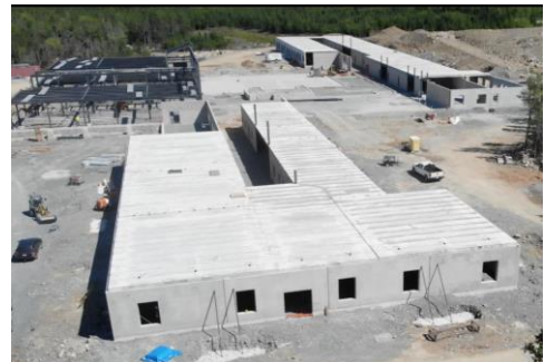
Construction progress of pre-cast panels and structural steel
